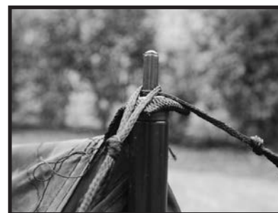
Step 6 - Place the looped end of the rope and slip over the pin on top of the pole.
