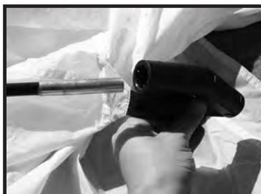
**Step 2 - Assemble the roof poles (B & C) and insert into the small opening of the molded joints.**
