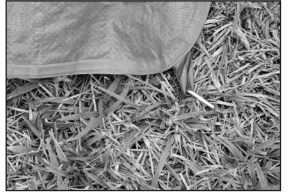
STEP 14 - Stake out the mud mat at the 2 corners.
